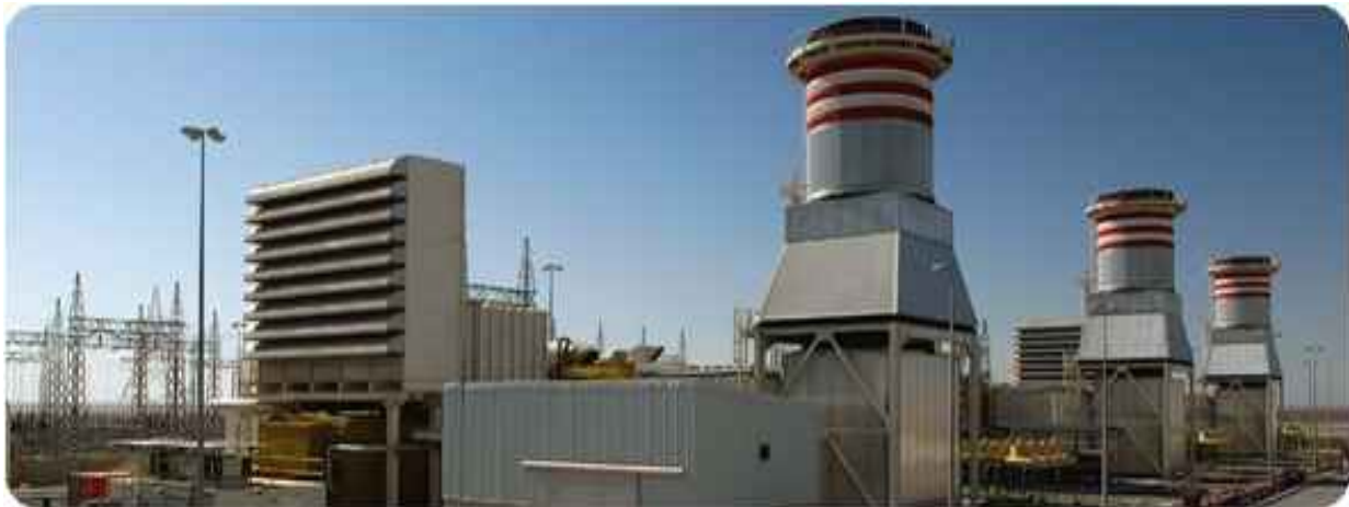
AL-KAMIL POWER PLANT - OMAN
